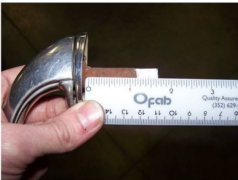
Fig. 1 Measure (Coupe) 1 3/4" or (Tudor) 1 7/16" from base with no gasket. Mark and cut shaft. If you are using a gasket you will need to add the gasket thickness to the length of the shaft.
